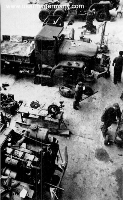
Left, 88th Maintenance Company Automotive Maintenance Platoon reconditions 5-ton trucks in open bays. Each of the five squads work on two or three trucks at a time. Below, soldier uses a cutting torch to free a stuck tow pintle. Below center, Sp4 Dana Howe spray paints a truck as one of the final steps. Bottom, Sp4 Gloria Maynard overhauls a vehicle transmission.
